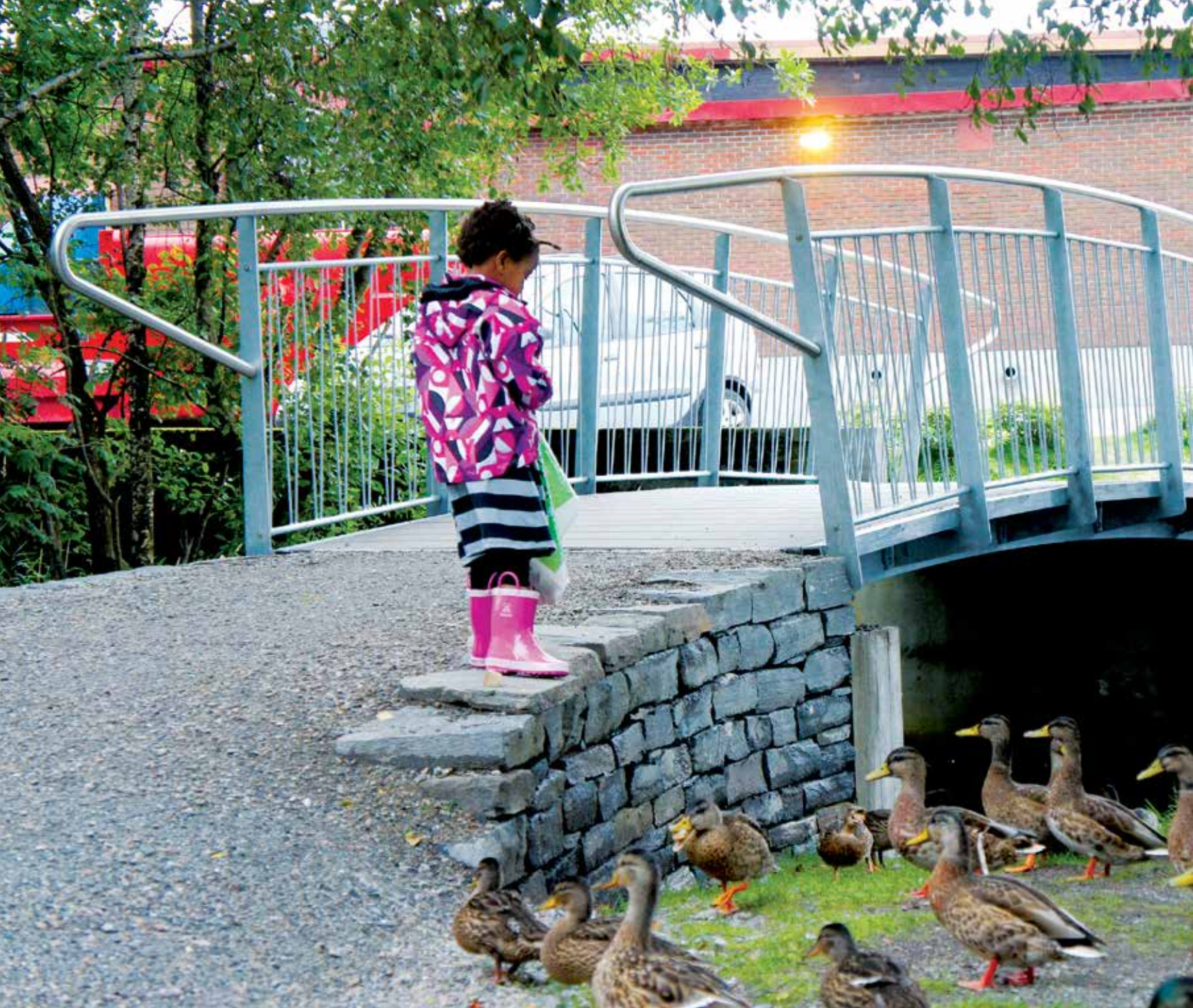
This Shortline Bridge with ZigZag fence has been installed in Bergen (NO) to provide access to a local park. One bridgehead has been elevated to create an attractive connection to the bank.
