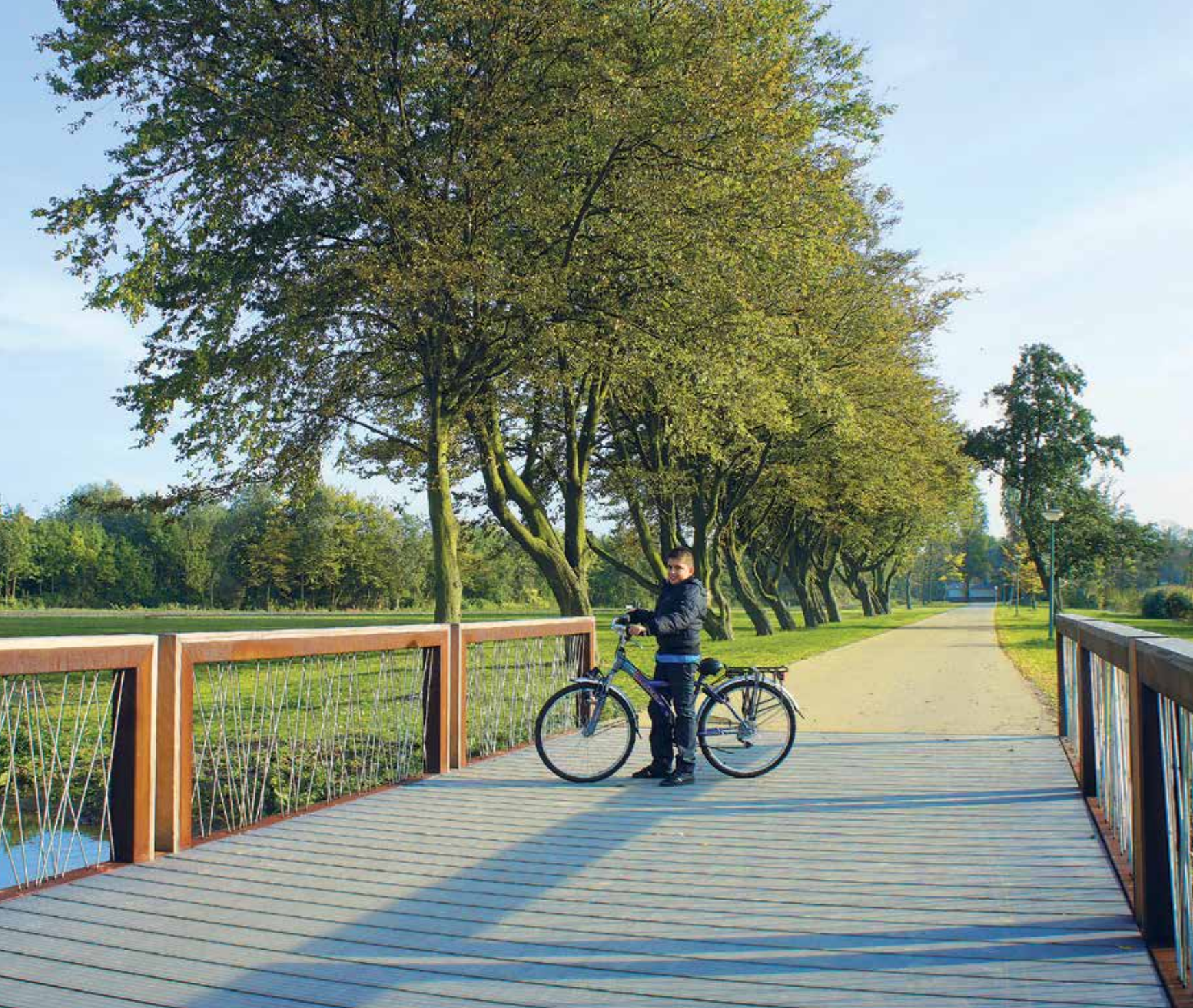
This stunning Crossline CorTen Bridge can be found at 't Nieuwelant Park in Vlaardingen (NL). The robust CorTen fences with criss-crossed balusters blend in harmoniously with the row of multi-stemmed trees!
