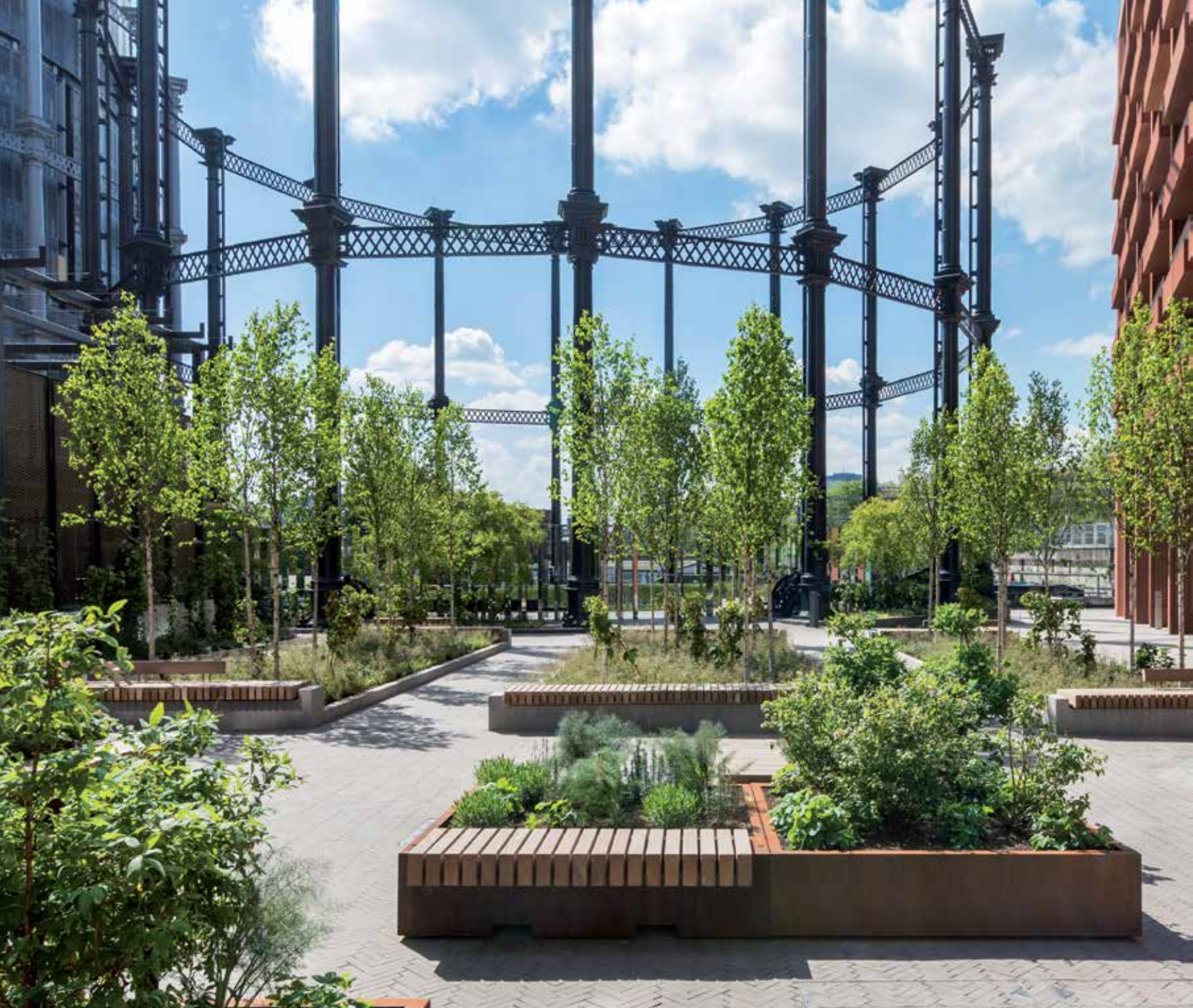
In recent years these gasholders in London have been redeveloped to become a sought-after real estate location. The outdoor space between the residential blocks features green islands of linked Big Green Benches and stone borders with R&R Top Seats.
